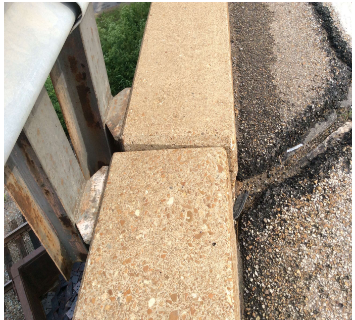
PHOTO 2 Description Left curb at Span 2 is out of alignment 1.5"
