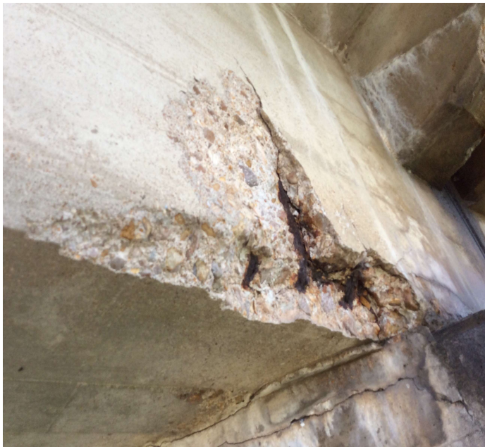
PHOTO 1 Description Spalls with rebar exposed to Girder 1 @ beginning of Span 2.
