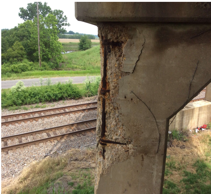
PHOTO 3 Description Spalls with rebar exposed to Column 1 @ Bent 1.
