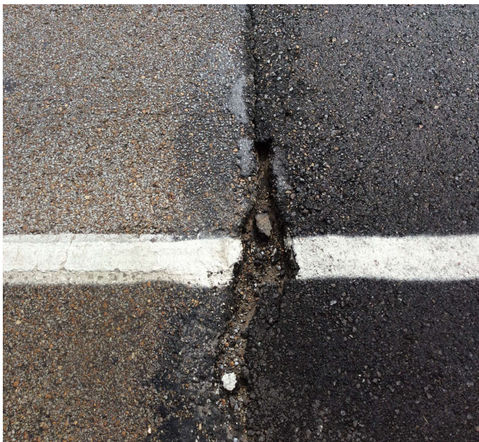
PHOTO 1 Description Pothole in deck in Left lane over Bent 1.
