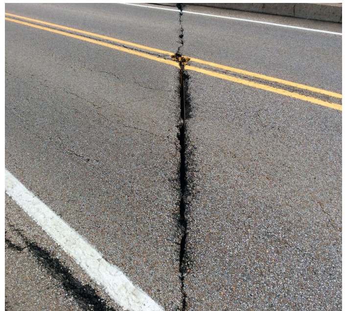
PHOTO 2 Description Spalls in asphalt @ joint @ end of Span 2.
