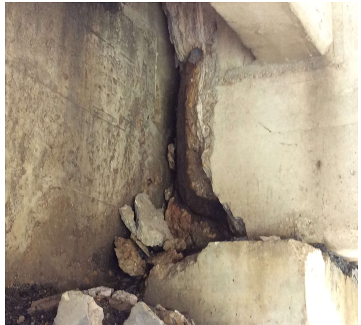
PHOTO 2 Description Spalls with rebar exposed to Girder 2 @ beginning of Span 5.
