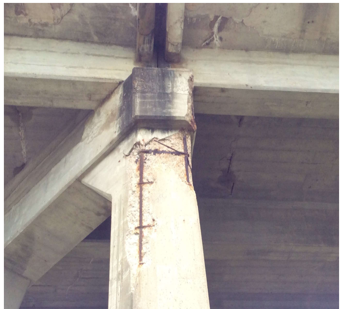
PHOTO 2 Description Spalls with rebar exposed to Column 3 @ Bent 4A.
