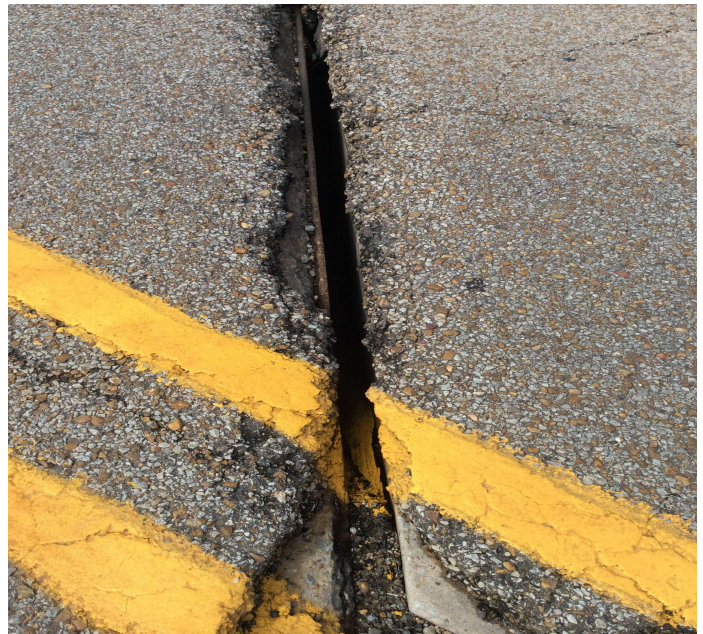
PHOTO 2 Description Joint seal over Bent 2.
