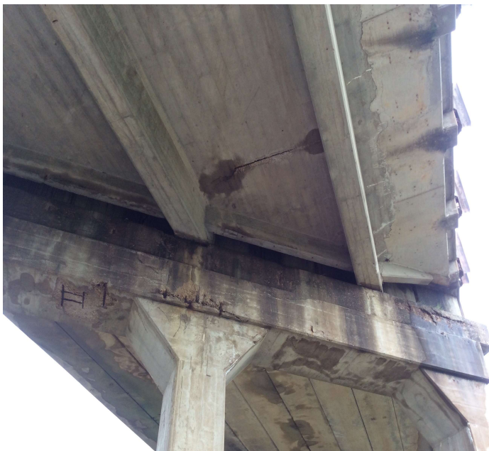
PHOTO 1 Description Spalls with rebar exposed to Cap @ Bent 3.
