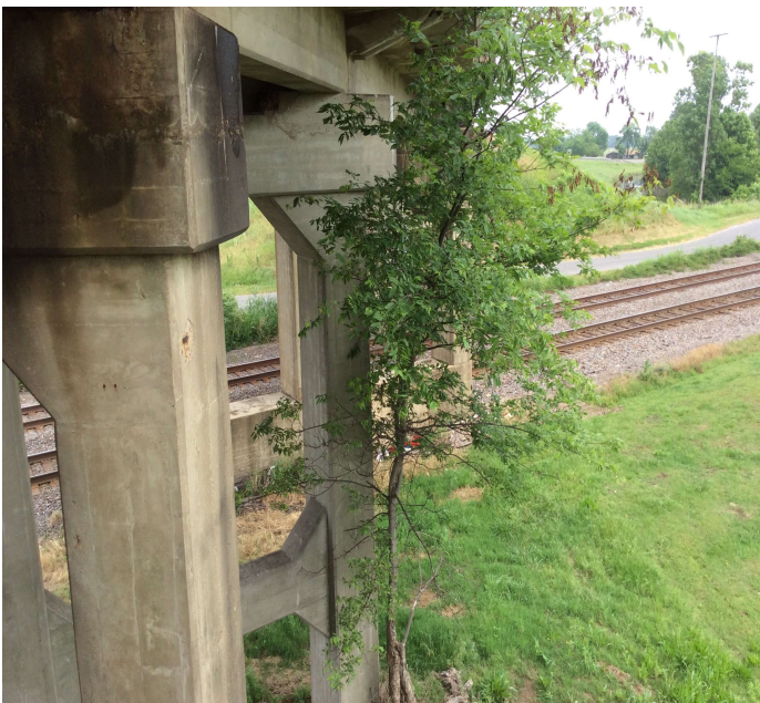
PHOTO 1 Description Vegetation @ Span 1.
