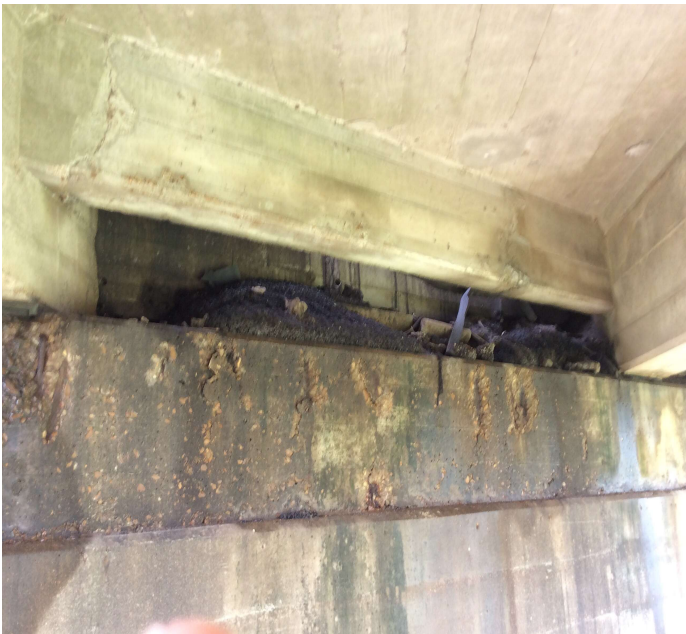
PHOTO 1 Description Debris on top of Cap @ Bent 2.
