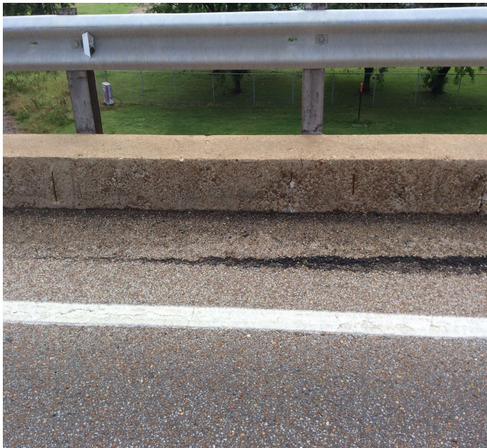
PHOTO 1 Description Spalls with rebar exposed to Right curb @ Span 3.
